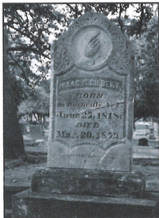
Left: Repaired headstone of Isaac Newton Gilbert. The die, broken into several pieces, was rejoined and securely mortared into the keyway of the base plinth.
