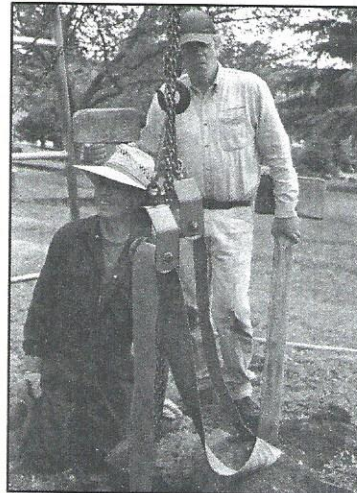
Grant Rutherford (right) supported Dale Palmquist in operating the chain hoist to lift a massive headstone element into upright position.
