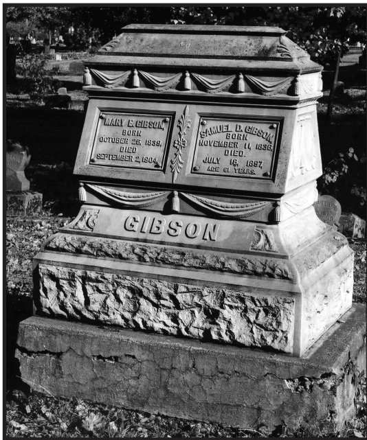
The grave marker of Samuel D. Gibson (1836-1897) and his wife, the former Mary Ellen Hiron Foreman, exemplifies the cast zinc monuments in Salem Pioneer Cemetery. Casting the metal from molds allowed elaboration that rivaled the crispness of stone carving.
