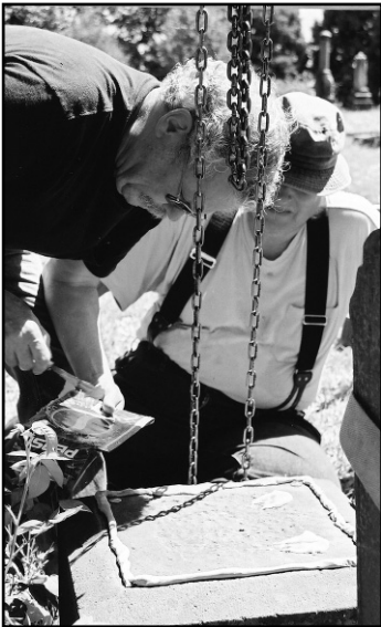
Mark Fields applied adhesive compound to rejoin a stacked monument in the Kurtz family plot in May while Fred Klatz observed the approved technique.
